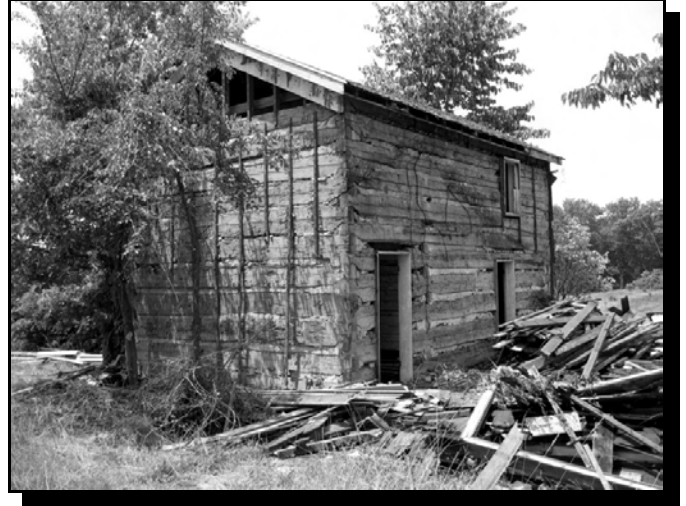
Rear view of the White log house, which has its original shake roof.
