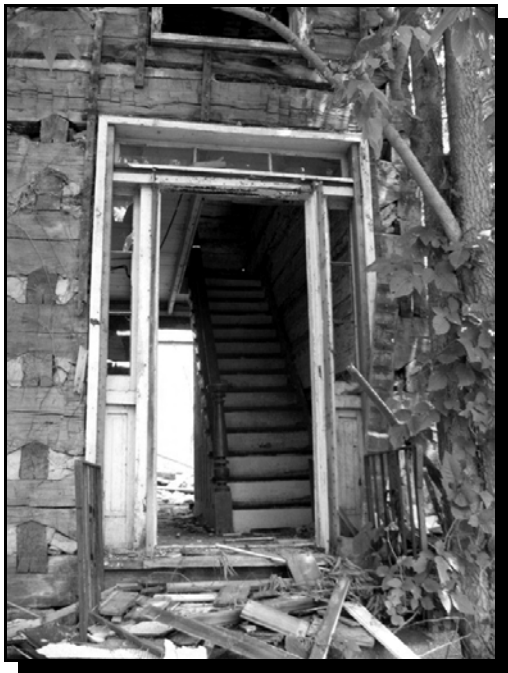
The distinctive Greek Revival entry of the c. 1840 White log house
